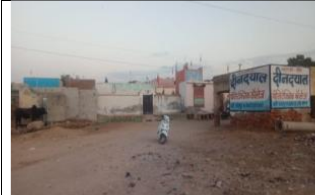
SPS near Railway Track
