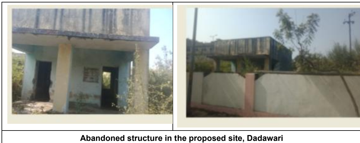
Figure 2: Photo of Abandoned structure in the proposed site, Dadawari
