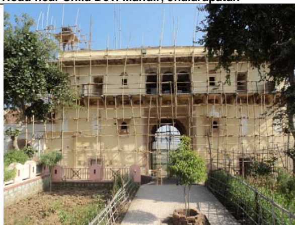
Heritage works under RUSDIP Project in Naulakha Fort, Jhalarapatan
