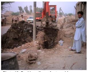
Photo 18: Backhoe digger for trenching
