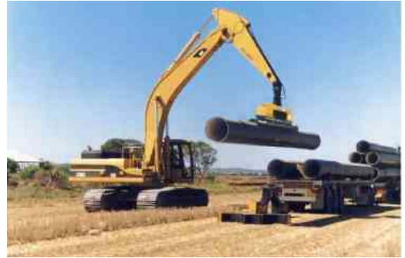
Photo 16: laying of pipeline using crane
