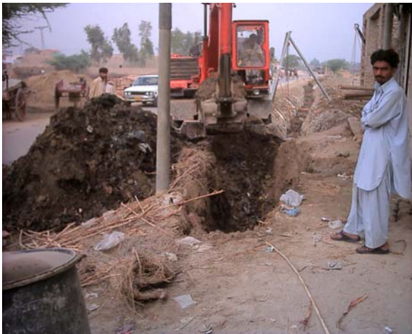
Photo 14: Back hoe trenching
