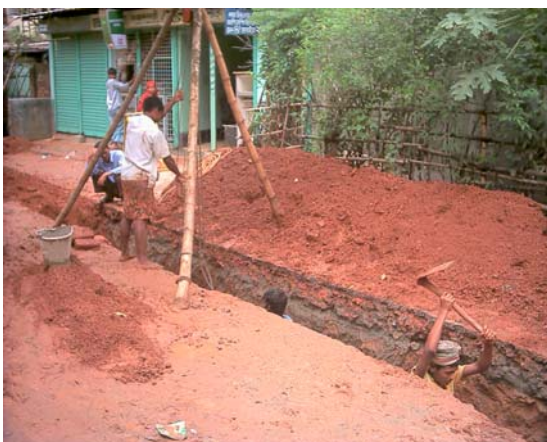
Photo 15: Digging a trench by hand
