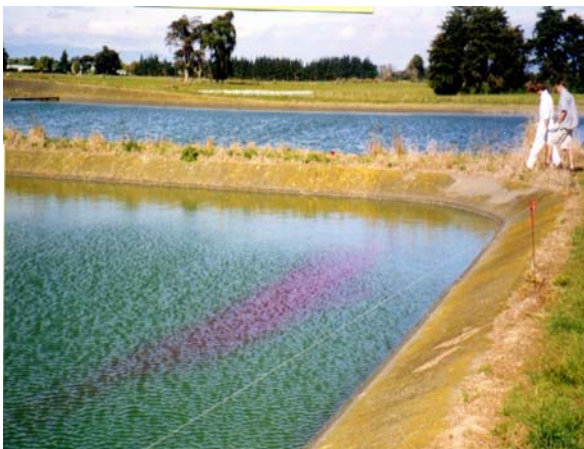
Photo 3: Typical STP Pond
