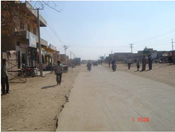
Photo 13: Enough space along roads for sewers
