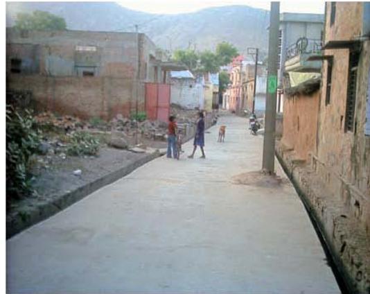
Photo 15: Roadside drains in Alwar
