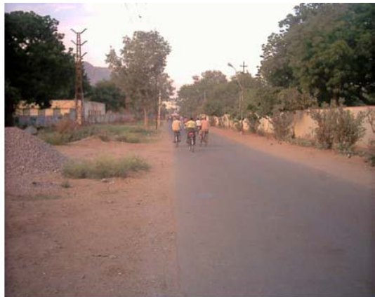
Photo 16: Road in the outskirts of Alwar
