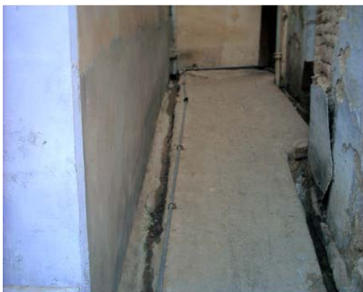
Photo 14: Above ground water supply pipes
