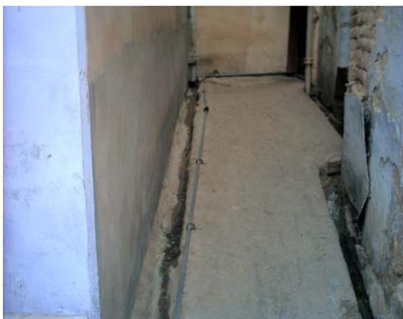
**Photo 8: Above ground water supply pipes**
