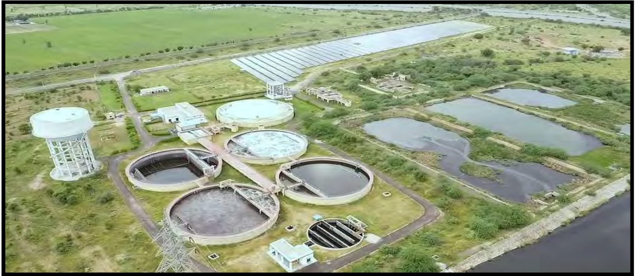
40 MLD STP at Bikaner
