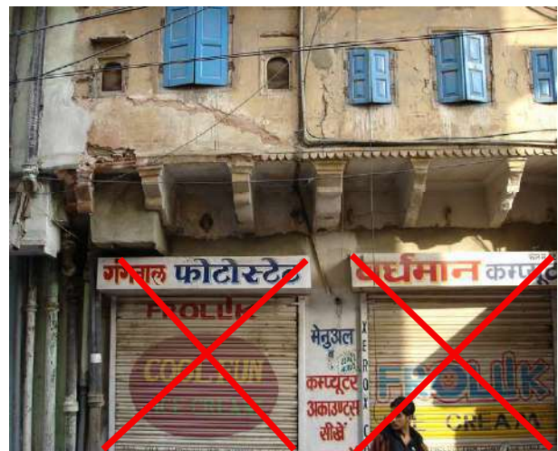
Restoration of modified openings
