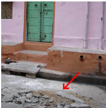
Repair of plaster/paving
