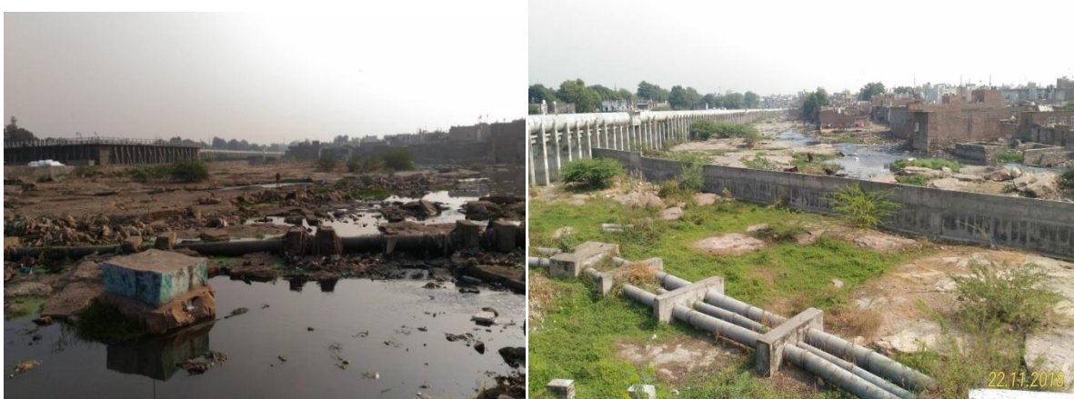
Mixing of STP outlet with untreated effluent
